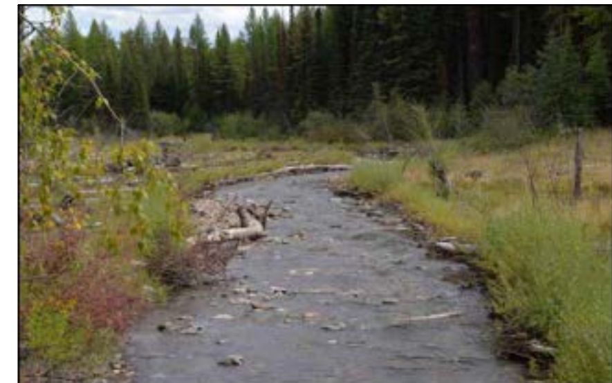
TYPICAL CONSTRUCTED STREAMBED THROUGH A RIFFLE FEATURE
