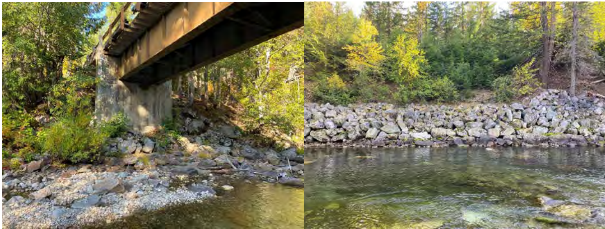
Figure 6. Left: Riprap material around the Little Wenatchee Road bridge crossing in Reach 6. Right: Riprap bank on river-left upstream of the bridge crossing in Reach 6.
